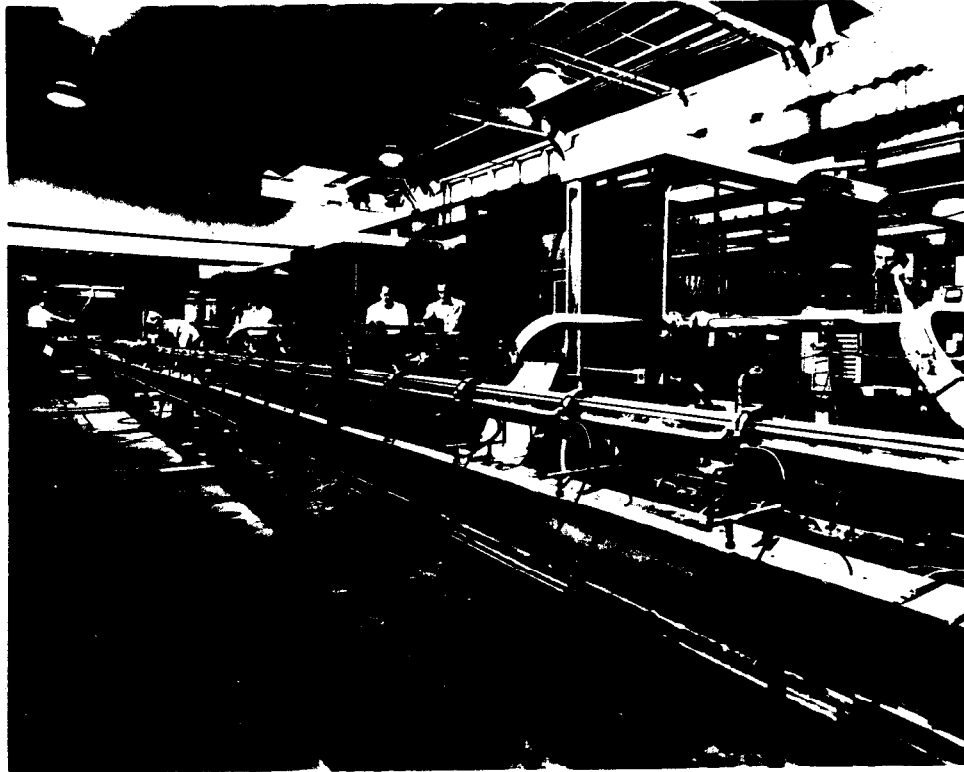
FIG. 22--The first sections of the Mark III accelerator, as seen looking in the opposite direction to beam motion (looking toward the injector). The twisted waveguide delivers power from the klystrons to the accelerator tube which is supported by the I-beams. After construction, the accelerator and I-beams were surrounded by concrete shielding.
