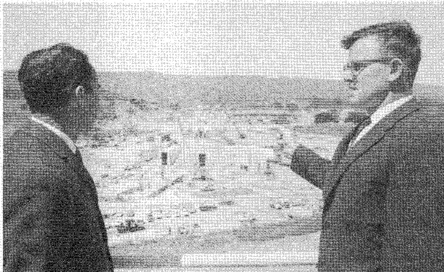
Doug Dupen (right) looks over construction of the center's beam switchyard with Stanford News Service writer Bob Lamar, 1965.
